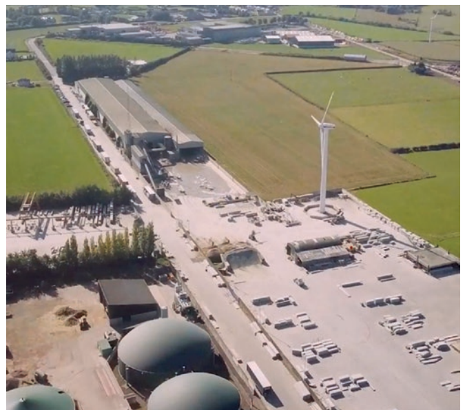
Aerial view of Creagh Concrete production site
